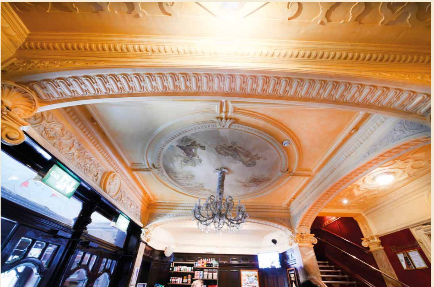
The Main Foyer which required cleaning and decorative repairs together with the carefully retouched artwork.
